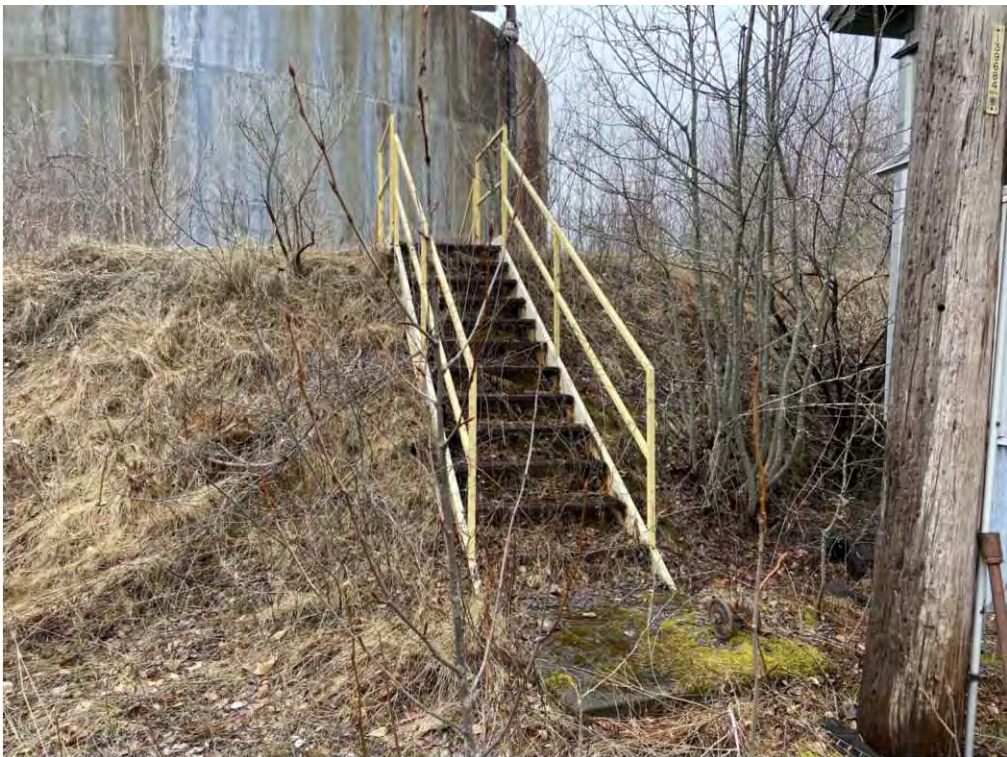
7 STAIRS OVER CONTAINMENT BERM C2.00 NOT TO SCALE
